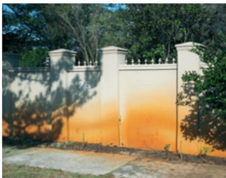
Figure 173. Iron and concrete (green) storm drain (above) and iron-stained garden wall (below).
